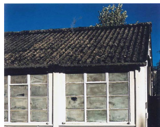
Asbestos cement roof
